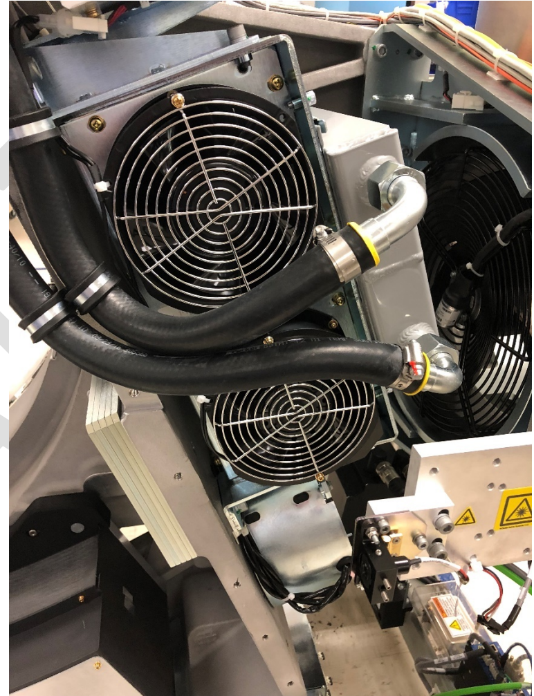
Figure 48 – Heat Exchanger Fans
